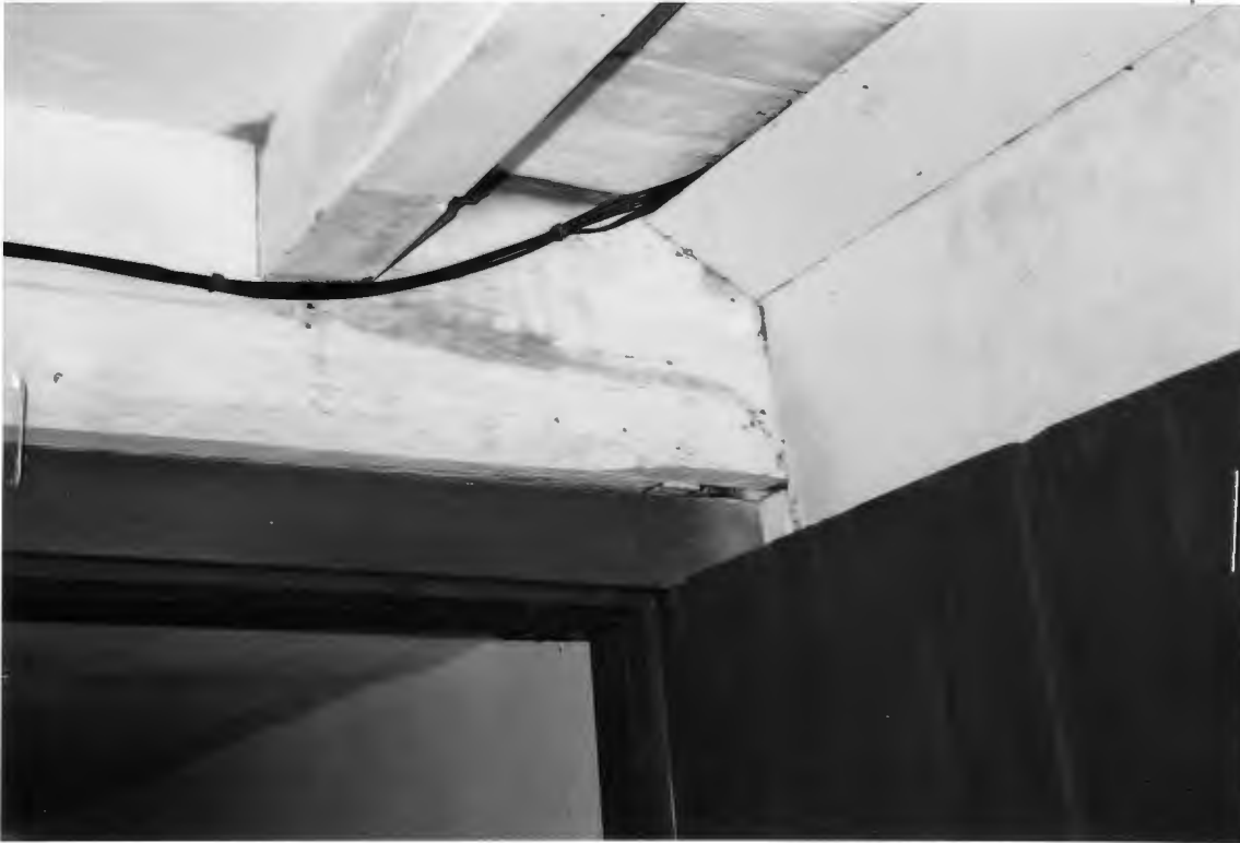
EAST GIRT/CHAMFER ↗ IN SW ROOM (ROOM 1)
