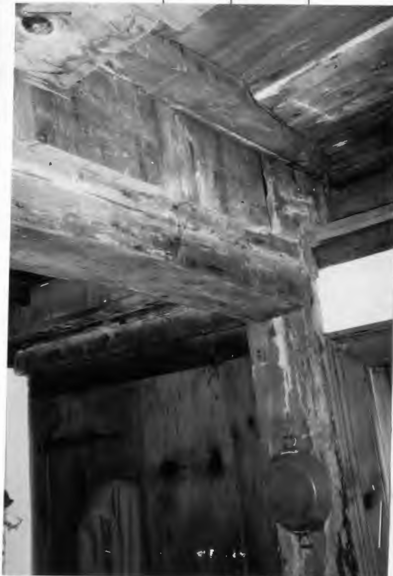
ORIGINAL END GIRT, CORNER POST AT NORTHEAST ADDITION - LOOKING NORTH
