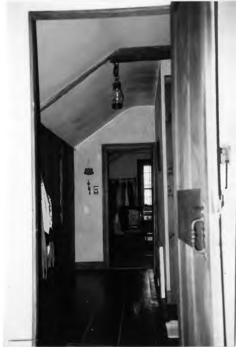
2ND FLOOR HALL - NORTH OF ATTIC STAIR VIEW CAST FROM BATHROOM ABOVE ROOM 3
