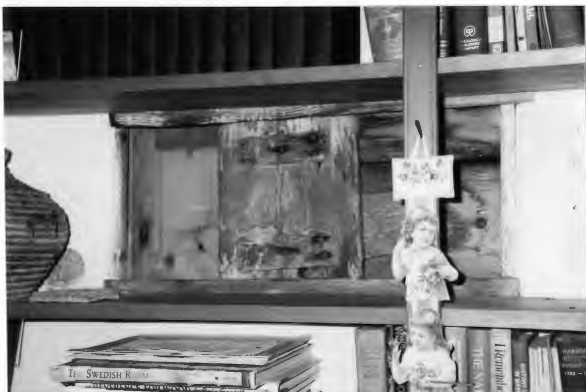
"OLD" WINDOWS/ SHUTTER AT SOUTH END OF ELL
