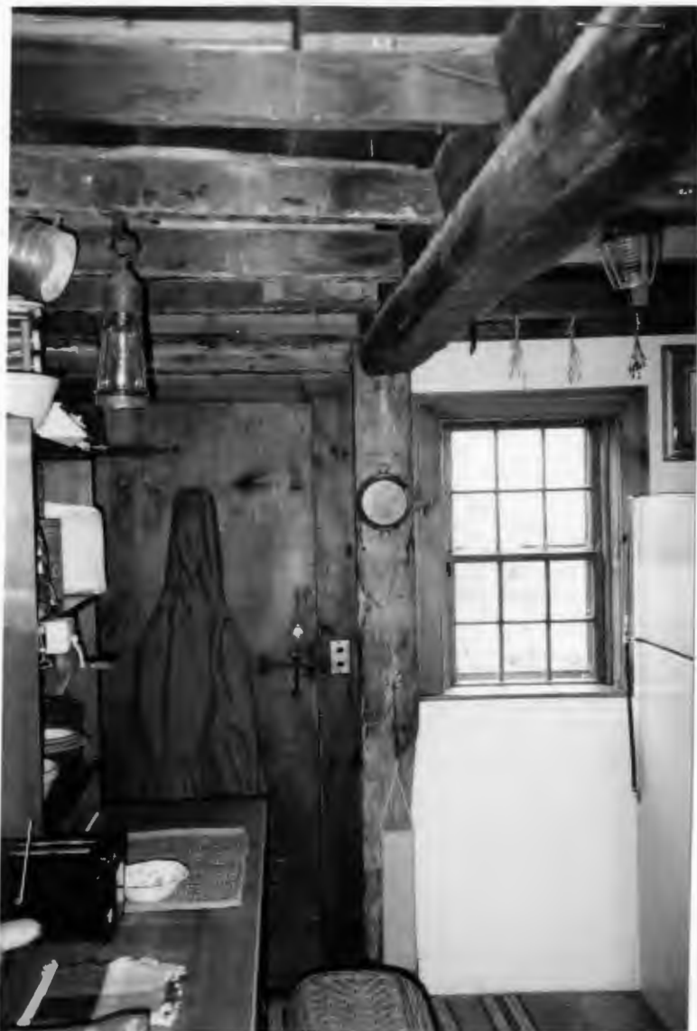
ROOM 5 - LOOKING NORTH (ORIGINALLY END TIE BEAM/ CHAMFER ON WEST SIDE ONLY)
