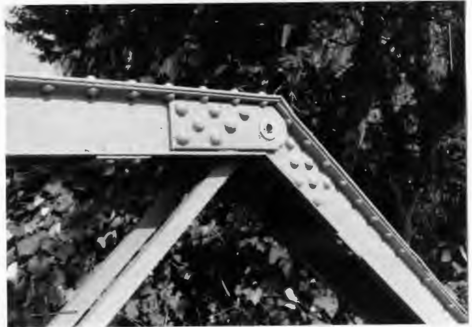
W TRUSS, N HIP, FROM SE
