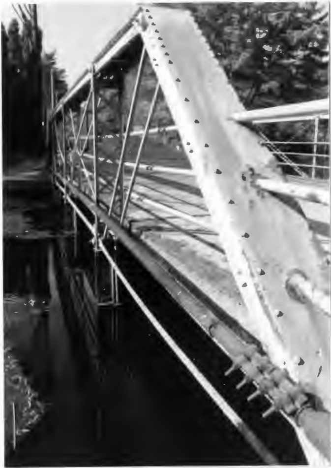
E TRUSS FROM NE
