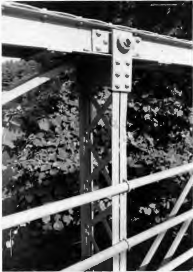
W TRUSS, NORTHERN INTERMEDIATE VERTICAL, FROM SE
