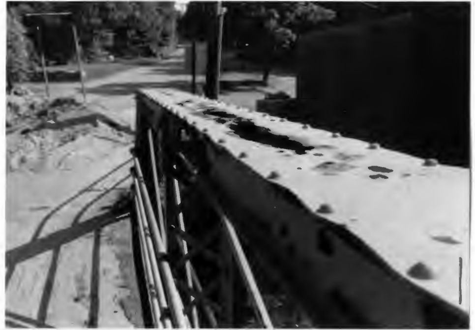
E TRUSS, NORTHERN END OF UPPER CHORD, FROM SW
