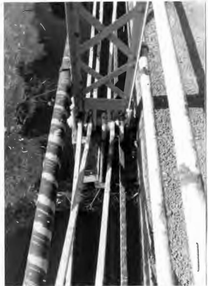
EAST TRUSS, CENTRAL VERTICAL. AND LOWER CHORD, FROM N
