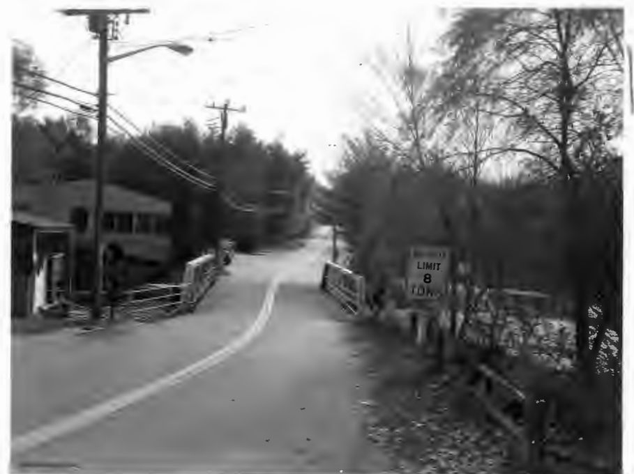
THRU VIEW LOOKING SE
