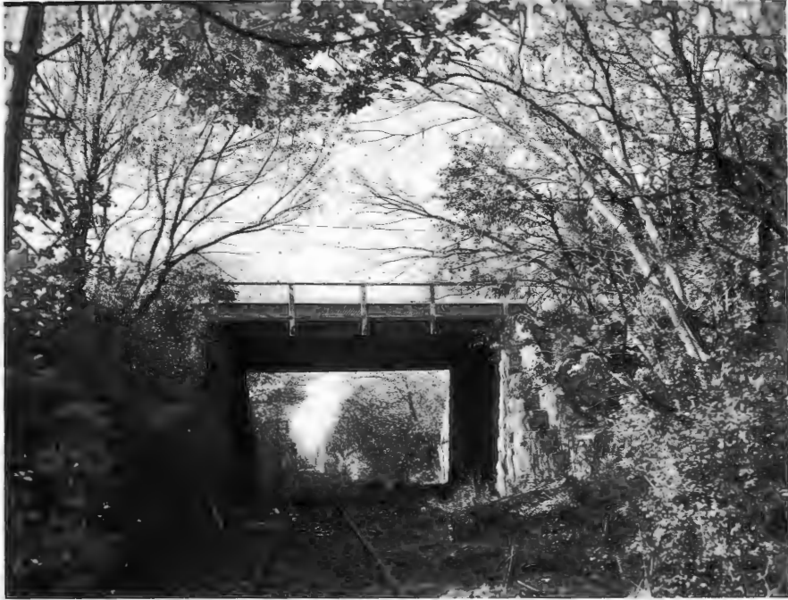
ELEVATION LOOKING WEST
