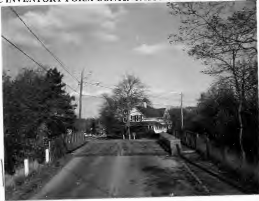
THRU VIEW LOOKING NORTH
