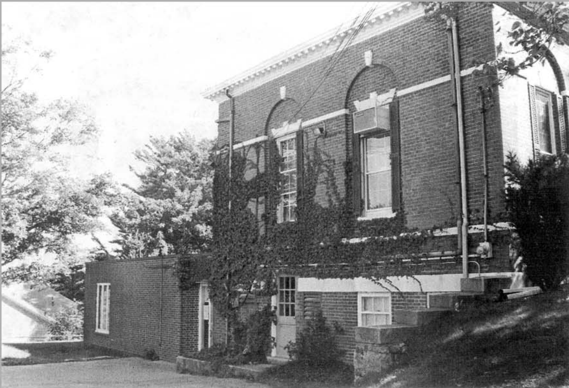
4. North façade, including 1965 addition, facing SE ( Photocopy ) (Photographer: Marilyn Fennollosa, 2000)
