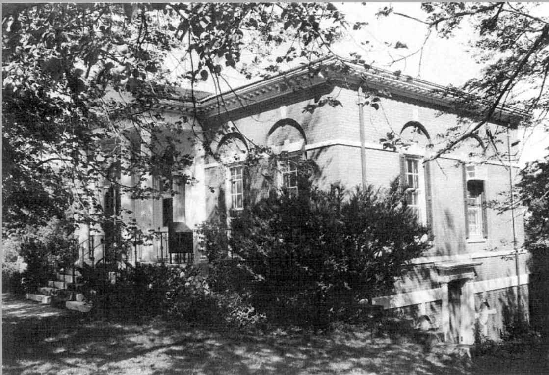
3. West façade, south façade, facing NE ( Photocopy ) (Photographer: Marilyn Fennollosa, 2000)
