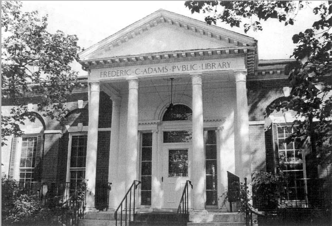
1. Front façade, facing E ( Photocopy ) (Photographer: Marilyn Fennollosa, 2000)
