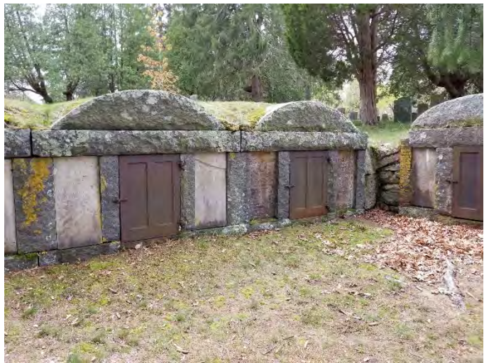
The five private tombs are built into the burying ground's north slope. While the interiors are materially sound, portions of the stone and brick work have deteriorated or failed.
