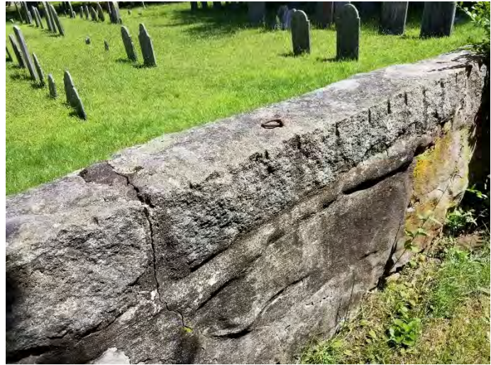
A parged granite block wall separates the burying ground from Main Street on the west side of the Church.
