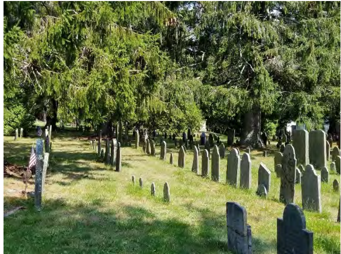
The Old Burying Ground is dominated by slate markers, many of them carved by local artisans. Many show signs of deterioration, including delamination, tilting, and breaking into fragments.
