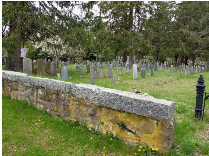
Granite block walls line both the east and south cemetery edges and portions of the walls act as retaining structures. Despite the age of the walls, they appear plumb, with only cosmetic deterioration.
