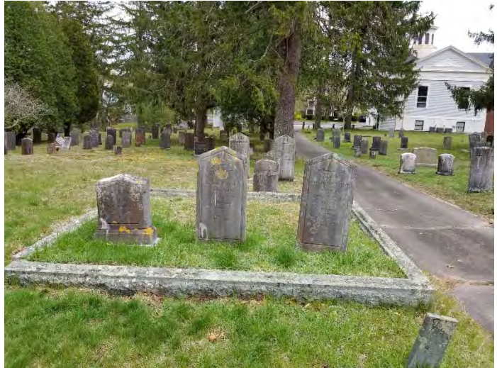
Granite curbs outline the edges of seven family plots within the burying ground, and several have begun to overturn. Build up of water in the soil and inadequate foundations are two likely causes.
